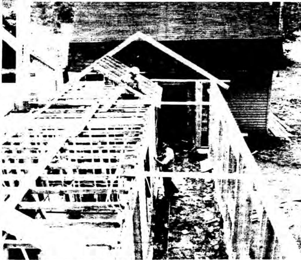
*View of connector under way; note roof framing of existing Shower Building and new connector.*
