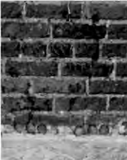
Photo 5. Interior plaster was removed from the lower 3 1/2' of the first floor interior to help the walls of the René Beaugard House dry out. Note the continuous layer of cement grout that has been installed in overlapping 1 1/4" holes that were drilled through the 16" thick walls. The large masonry columns were also dampcoursed to stop moisture from deteriorating the replaced cyprus porch beams above. Photo by Douglas Hicks, Williamsport Preservation Training Center, NPS.
