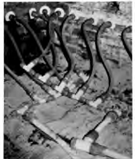
**Photo 8.** After the rotted floor joists were removed and the crawl space cleared of debris, holes were drilled about 5' apart and chemical resins (a silicate compound with aluminum stearate in an alcohol base) were injected into the brick walls. The chemicals flood the porous mortar and bricks and upon curing form a moisture proof dampcourse layer. To date, this chemical layer appears to be effective. Photo by Southeast Regional Office, NPS.
