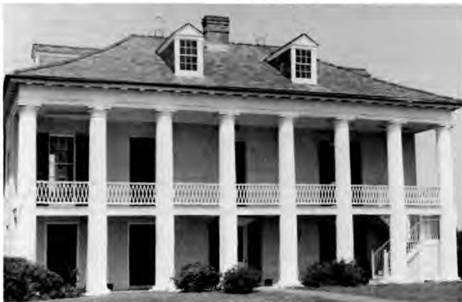
Photo 4. The René Beauregard House, ca. 1830, suffered from rising damp due to the high ground water adjacent to the Mississippi River. In 1979, a dampcourse layer of cement grout was installed at the base of the building. Stucco repair to the exterior cosmetically covered the visually disfiguring drilled holes. Photo by Douglas Hicks, Williamsport Preservation Training Center, NPS.
