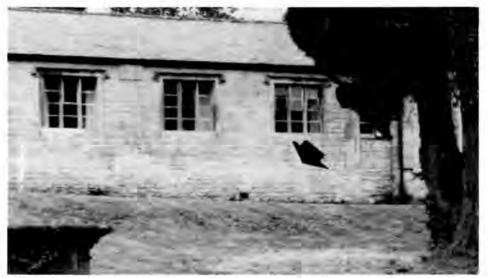
Photo 1. Rising damp is seen along building foundations as a tidemark three or four feet above grade. This tidemark differentiates the wet from the dry area of the foundation wall. Rising damp is generally found in low lying or moist areas.
