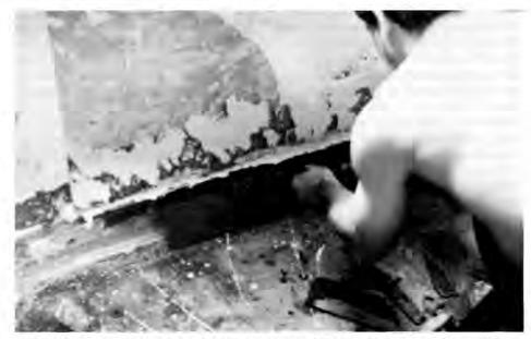
Photo 2. New dampcourses can be mechanically cut into foundation walls. In this regularly coursed brick wall, a heavy polyethylene sheeting is being installed in a slot that has been cut with a tungsten carbide saw. Slate shims and non-shrink mortar are used to hold the sheeting in place.
