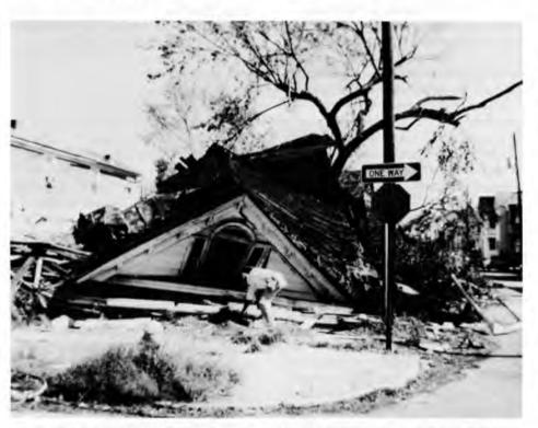
This house collapsed as the eye of the storm came in the direction of the "one way" sign shown in the picture. The walls fell from under the roof framing although the roof structure remained basically intact.
