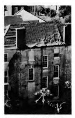
Puckered metal roof. Although the roof is still intact, the cleats were probably sheared.
