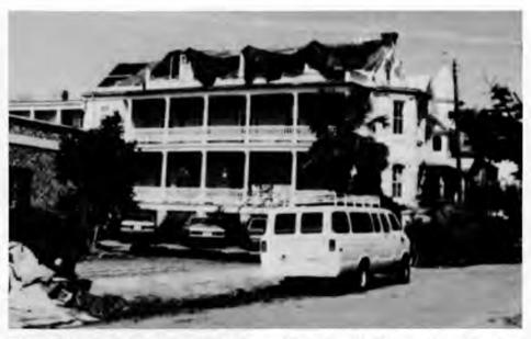
The immediate reaction to roof damage was to throw up plastic or canvas tarps to cover destroyed areas and to help prevent further interior damage.
