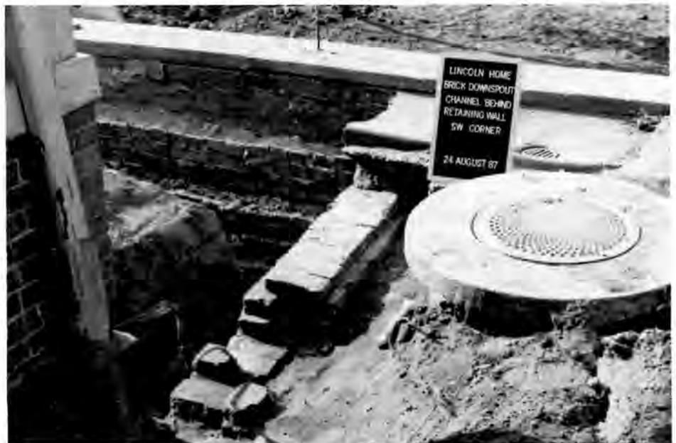
Remnant of a drainage channel discovered behind the Lincoln Home front yard retaining wall during the 1987 restoration. The drain, which dates from the 1850s, carried rainwater from a downspout through the retaining wall. Photo by Vergil Noble.
