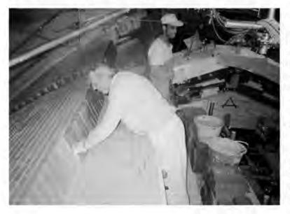
(0°,  $\pm 45^{\circ}$ , 90° angle ply) tissue of aramid fibre of 230gr/m<sup>2</sup> is glued using epoxy resin.
