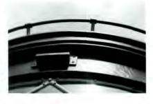
(Below and top right) Close-up of the deteriorated conditions of Anacapa Island Lighthouse before rehabilitation and finished metal work on the lantern after rehabilitation. Photos courtesy USCG. hacapa Lighthouse is located on Anacapa Island, 11 miles off the coast of Port Hueneme, California. Built in 1932, it was the last lighthouse built by the U.S. Lighthouse Service. Until the 1995-1996 Coast Guard rehabilitation, Anacapa Lighthouse had never undergone any major repairs.
