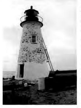
softer and more friable than that of the exterior; the joint repairs made by the lighthouse keeper(s) over the years were most likely exterior rather than interior. using more portland cement as it became available. Analysis of the inside mortar reveals only lime and sand, with bits of hair and other materials; no oyster shell was noted. The U.S. Coast Guard Lighthouse Maintenance Reserve Unit has offered their services to the U.S.
