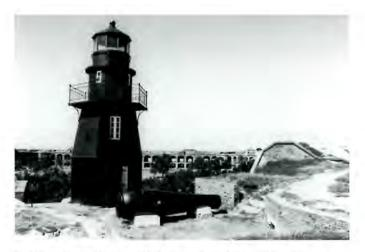
The Tortugas Harbor Lighthouse (1876) was constructed of wrought iron because a brick structure on the wall of the Fort would create dangerous fragments if hit by an exploding shell. Photo by Ralph Eshelman, 1996 courtesy NPS.
