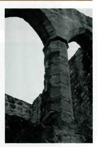
structure were retained, but the internal partition walls were demolished and replaced. All of the new masonry was laid in lime mortar, with the exception of the drums of an octagonal column, which were laid in gypsum mortar. These rebuilt elements of the convento were meant to serve as interior spaces, with the column accenting the second story of a stair hall; however, in 1868 the Column condition before restoration, detail, 1992.
