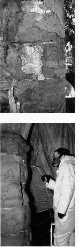
Applying consolidant to column surface. HS203A-North wall, 1993. Benedictines were forced to abandon the site, and the convento was never roofed.
