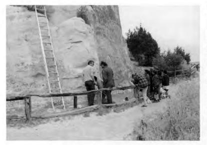
Conservation team evaluating stone deterioration along the trail. Photo by Scott Kreilick. is probably accelerated due to surface drying resulting from windy conditions. Disintegration may be due to the dissolution of clay rims, which are the principal form of cement in this particular strata.
