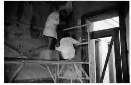
cases where removal would seriously compromise the historic plaster. It was replaced with more sympathetic material made of hydrated hydraulic lime and sand. Deep losses within the plaster body were filled with edging material and recessed approximately 1/8" below the fragment surface. Shallow fills and open cracks were filled with a mixture of one part hydrated hydraulic lime and three parts fine silica sand.
