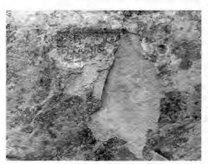
breaking off of pieces of the rock; the removal, grainby-grain of the sandstone by weather: the effects of lichens and micro-flora growing on the rock, such as by the physical prying of their roots and the rock-dissolving chemicals that they excrete: and the deposition of fine, clayey materials that are washed down the face from the mesa top and which dry and harden on the face,
