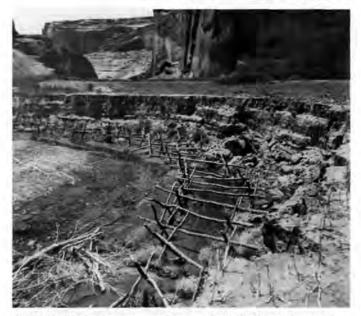
Oak "spider" jetties down stream at junction of Twin Trails and Canyon del Muerto installed in 1951 in order to stabilize active streambank erosion. Nothing is left of the jetties installed along this 300' stretch of streambank, 1951. Photo by Paul Balch.
