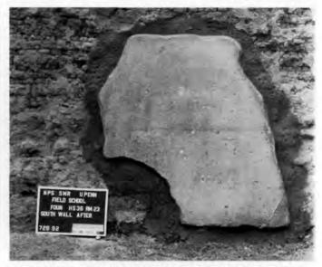
Fig. 8. Mechanics Corral (HS 36), Room 23, Fort Union. Plaster fragment after recent conservation. Note new edging flashed into adobe wall.
