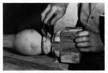
Fig. 2. This deteriorated baluster was removed for careful conservation and reinstalled during the 1970s restoration of the Morse-Libby Mansion, Portland, ME. Photo by Morgan Phillips.
