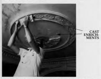
Fig. B. Ornament layout is determined using plane geometric principles; segmented locations are deeply scratched to provide a rough surface for adequate bonding using plaster as an adhesive. Photo by Peter Sanders.
