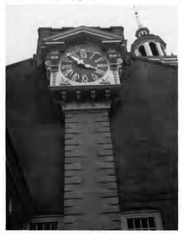
Fig. 8. Independence Hall's Reconstructed Clock (1972-73). Cast stone and wood with fiberglass and polyester bronze ornamentation. Photo by Lee H. Nelson, FAIA.
