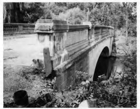
Fig. 1. Deterioration of deck, parapet wall and efflorescence. Photos by LANDSCAPES.
