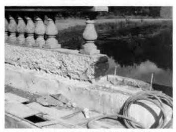
Fig. 2. Removal of unconsolidated concrete and portion of parapet in section of lost balustrade. Photo by LANDSCAPES.
