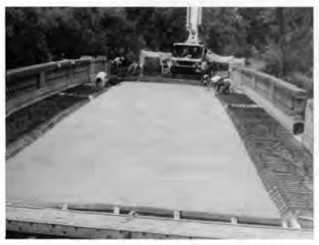
Fig. 4. Deck pouring underway with the rebar for new sidewalks in place. Photo by LANDSCAPES.
