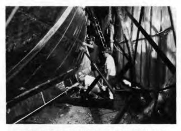
*Snow Squall* project director David Switzer, maritime intern Karl Bodensiek, and HAER Architect Dale Waldron (from left) attach station lines to the bow section of the clipper ship in preparation for measurement of the hull's starboard side curvature. Photo by Molly Horvath, 1992.
