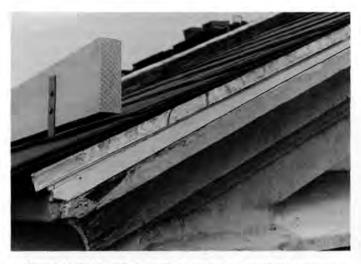
6. Cypress, a durable wood, was selected for the snow boards and stainless steel was selected for the support brackets because it will not corrode. Note the lead coated copper drip edge under the slate and the slight kick-up at the eave created by a cypress wood spacer. The deteriorated portion of the cornice was in the process of being repaired.
