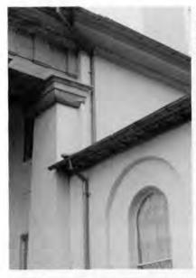
4. New gutters and downspouts repeat the historic configuration, but are slightly larger to handle water run-off. Note the elongated elbow on the upper section.
