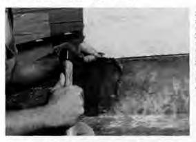
3. Traditional methods were used to pack lead wool into flashing reglet (narrow slit) joints to hold the cap flashing tight with the stuccoed chimney.
