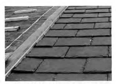
Modern methods of detailing joints were used where moisture could penetrate to the roof deck. At this offset between the lower portico roof and the main block, a hidden rubberized membrane was selectively used in connection with traditional lead-coated copper flashing.
