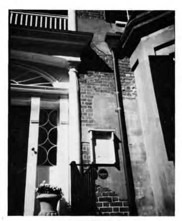
The existence of such fine quality mortar joints is evidence that this brick house in Charleston was not stuccoed originally.
