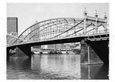
Smithfield Street Bridge (1883, 1891). Designed to span the Monongahela River in Pittsburgh by Gustav Lindenthal, one of America's most prominent bridge engineers, this is the oldest steel-truss bridge in the country. It is scheduled to be rehabilitated for continued vehicular use. Photo by Jack E. Boucher for HAER, NPS.
