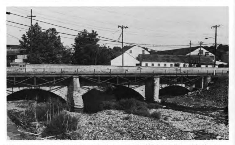
Main Street Bridge (1851, 1874). This stone bridge in Phoenixville, Pennsylvania, underwent its first rehabilitation in 1874. The unusual Fink metal trusses were added to carry a streetcar line. Current plans call for two 40-foot sections of the bridge to be used as a pedestrian bridge in a county park. Photo by Robert Vogel, Smithsonian Institution.
