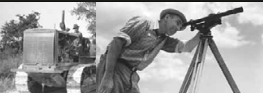
Far left: Enlistee grades a road in Mammoth Cave National Park, around 1935. Near left: Surveying for a new road for the Blue Ridge Parkway.
