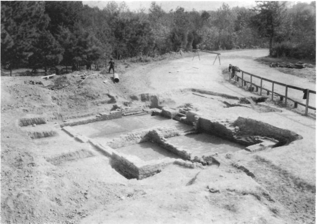
FIGURE 3 Excavation of a brick foundation (Unit A), Jamestown Island, 1936 (HABS VA,48-JAM,1-1. HABS/HAER/HALS Collection, Library of Congress)
