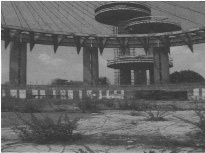
FIGURE 2 New York State Pavilion, Queens, New York, 2008. (Courtesy of the author)
