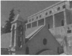
FIGURE 1 The Old English Hospital complex in the city of Salt is a prominent urban landmark. (Courtesy of the author)
