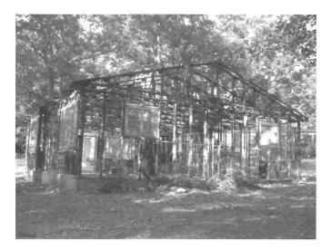
FIGURE 3 Disassembly of the Lustron house is in full swing as the crew removes the steel framing pieces supporting the chimney flue, and the crane lifts another whole roof truss off and over the shell of the house. (Courtesy of the authors)
