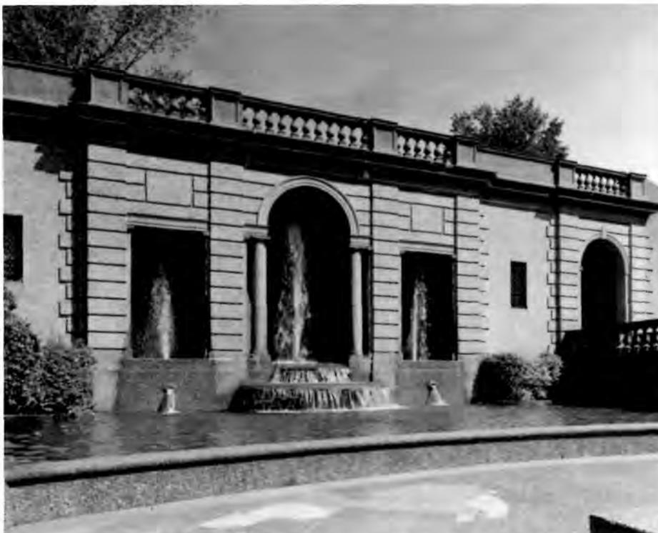
The great terrace not only serves as a focal point for Meridian Hill Park, but also as an immense retaining wall and design element for the water source of the cascade. Based on Italian Renaissance traditions, the central water jet serves as the spring source which cascades over 15 falls until finally settling in a large, peaceful reflecting pool at the base of the hillside. (Photo by Jack E. Boucher, HABS 1976)
