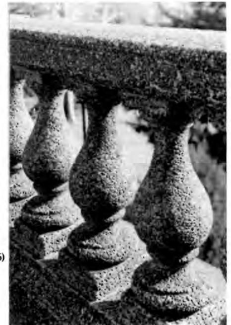
Meridian Hill Park served as a prototype for large scale and decorative usage of exposed aggregate concrete. Many areas in the park are showing considerable wear and the large format photography and measured drawings will assist in future maintenance of the resource. (Photo by Jack E. Boucher, HABS 1976)
