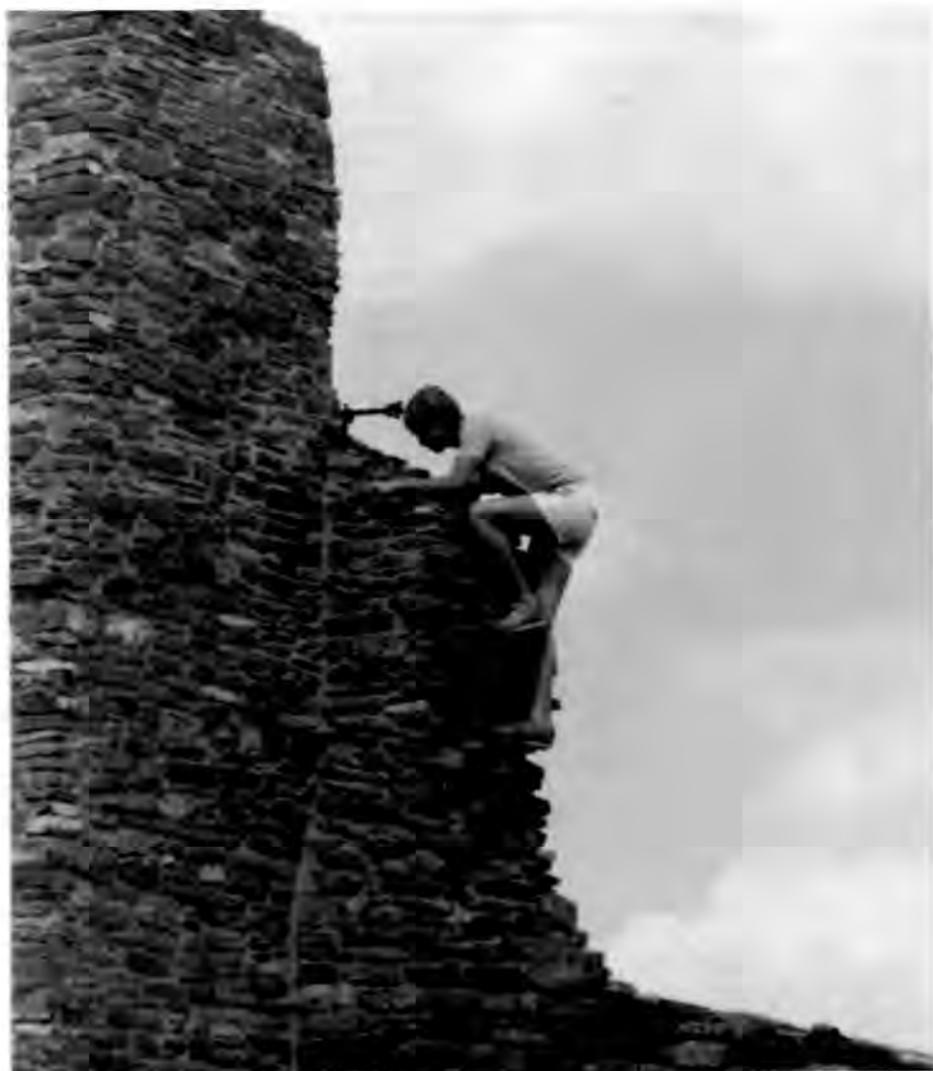
John Jennings scales a 40-foot wall at Salinas National Monument, NM with a vectron electric distance meter focused on a mirror at the end of the pole to provide a height reading. (Photograph by Rudd Long, 1985)
