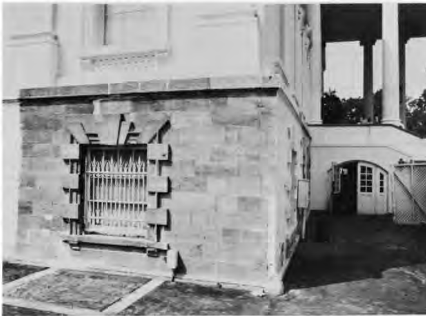
Test area B (see diagram to the left) after paint removal.
