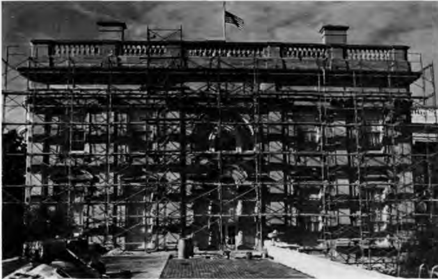
White House, east elevation with scaffolding, after paint removal.
