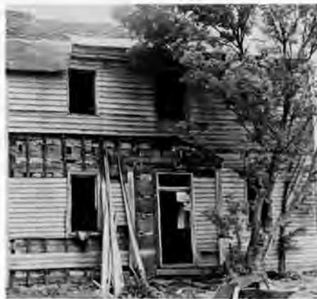
The Zachariah Price DeWitt log cabin built in 1804 in Butler County, Ohio, here awaits restoration. Not only has this 2-story house been incorrectly labeled as a "cabin," but it has been stripped of its siding, which, if not original, was probably applied soon after the building was constructed and was part of the history of the building. Photos: National Park Service Files.
