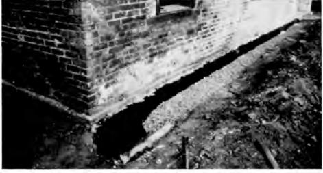
Photo 1. Whenever possible, ground moisture, wicking into a building, should be diverted from the foundation of a building. Shown is a sloped drain pipe, placed in a gravel bed at the base of the foundation wall. The below grade foundation wall has also been treated with a water-proof bituminous coating to retard lateral damp. The new drain will divert water away from the footing and relieve seasonal hydrostatic pressure. Photo by J. Stubbs, NPS.
