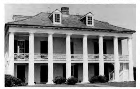
Photo 4. The René Beauregard House, ca. 1830, suffered from rising damp due to the high ground water adjacent to the Mississippi River. In 1979, a dampcourse layer of cement grout was installed at the base of the building. Stucco repair to the exterior cosmetically covered the visually disfiguring drilled holes. Photo by Douglas Hicks, Williamsport Preservation Training Center, NPS.
