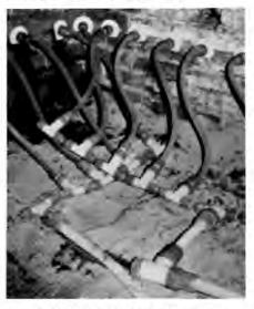
Photo 8. After the rotted floor joists were removed and the crawl space cleared of debris, holes were drilled about 5" apart and chemical resins (a siliconate compound with aluminum stearate in an alcohol base) were injected into the brick walls. The chemicals flood the porous mortar and bricks and upon curing form a moisture proof damp-course layer. To date, this chemical layer appears to be effective. Photo by Southeast Regional Office. NPS.
