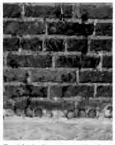
Photo 5. Interior plaster was removed from the lower 3½' of the first floor interior to help the walls of the René Beauregard House dry out. Note the continuous layer of cement grout that has been installed in overlapping ½' holes that were drilled through the 16" thick walls. The large masonry columns were also dampcoursed to stop moisture from deteriorating the replaced cyprus porch beams above. Photo by Douglas Hicks, Williamsport Preservation Training Center, NPS.
