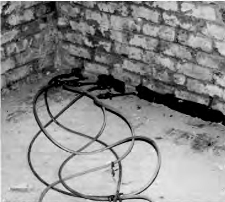
Photo 3. Chemically injected resins can also form a dampcourse layer in some buildings. Holes are drilled approximately every five inches along a masonry joint line or horizontally in the brick. In this case, the dampcourse is installed just above a slab-on-grade floor. The chemicals are injected under pressure, saturate the masonry and upon curing form a barrier to the rising damp.
