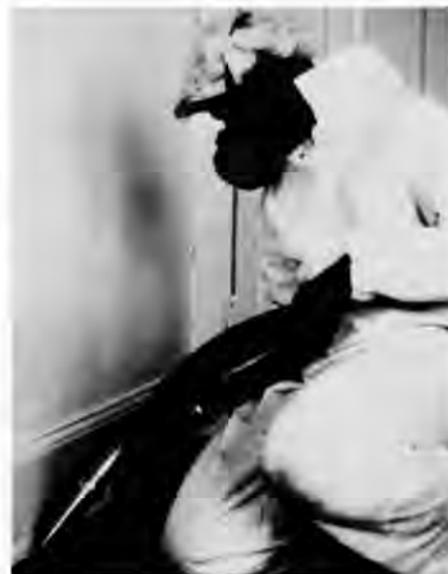
Workers should wear protective gear and specially designed respirators at all times during the abatement. Only high-efficiency particulate air filter vacuums (HEPA-vacuums) should be used as they prevent lead-laden dust from re-entering the abated space. Photo courtesy of the National Institute of Building Sciences and James Keck, Baltimore City Health Department.
