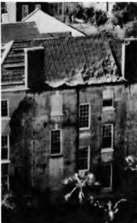
Puckered metal roof. Although the roof is still intact, the cleats were probably sheared.
