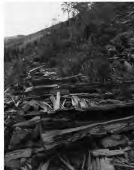
Granier ditch segment located along Rock Creek a few miles upstream from Atlantic City. A rock wall was built to support a flume at a spot where the ditch crossed a steep hillside. Photo by Richard Collier, 1985.
