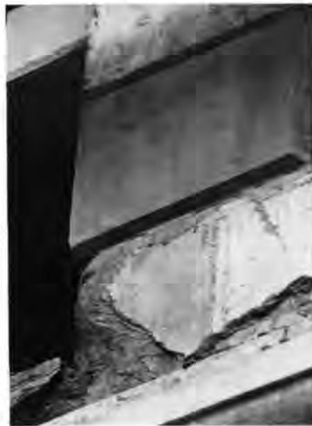
This photograph illustrates repair of historic sandstone using a composite patching method which involves patching the deteriorated portions of the stone with a cementitious material containing an aggregate of sand or crushed stone. Sometimes artificial coloring may be added in order to make the patch blend with the stone, or the patch can be painted to match the adjacent stone. Photos by National Park Service.
