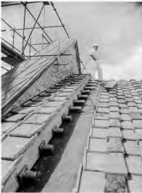
The cylinders that contain the special anchorages connecting the tympanum and the roof.
