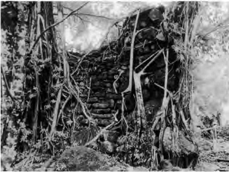
End wall of Kinyear Fulat on Leluh, Kosrae, Federated States of Micronesia. Banyan trees have colonized the wall and now serve as the principal supports within the wall structure; their roots pass through the wall and have gradually undermined the structural integrity of the wall itself. See Beardsley's article, page 51. Photo by Felicia R. Beardsley.
