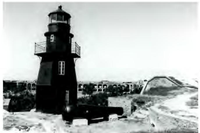
The Tortugas Harbor Lighthouse (1876) was constructed of wrought iron because a brick structure on the wall of the Fort would create dangerous fragments if hit by an exploding shell. Photo by Ralph Eshelman, 1996 courtesy NPS.
