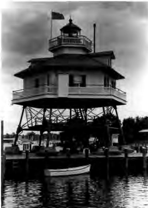
move of the lighthouse about two nautical miles to the museum's waterfront was accomplished in the spring of 1975. Fortunately, because a new bridge was being constructed nearby, the B. F. Diamond Construction Company of Savannah, Georgia, was in the right place at the right time. The seven, 10"-diameter, solid cast-iron piles were severed at the water line while a 110' boom, steam-operated crane placed on a barge lifted the entire three-story lighthouse and rested it on the side of a barge for
