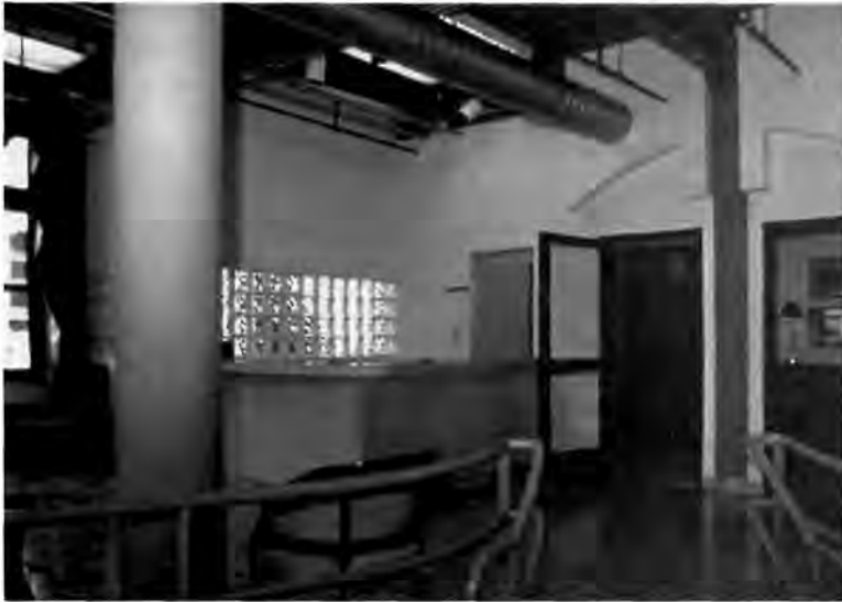
Exposed new mechanical and structural systems are compatible with industrial or warehouse conversions. Photo courtesy National Park Service.
