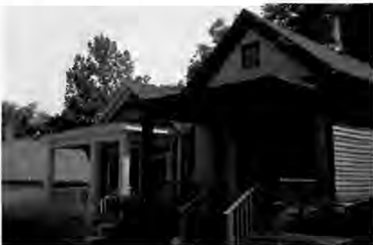
Rehabilitation of the shotgun houses in the Sweet Auburn Historic District of Atlanta, Georgia, created affordable housing. Photo courtesy Georgia Historic Preservation Division.
