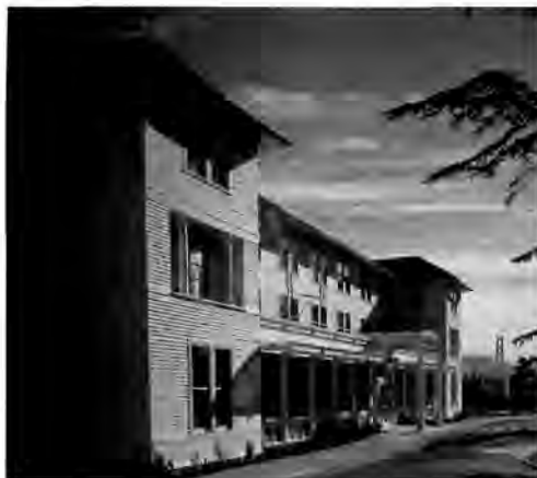
The Letterman Hospital Administration Building at the Presidio, San Francisco, is being rehabilitated for the Thoreau Center for Sustainability, using the Rehabilitation Tax Credits. Photo courtesy Richard Barnes.
