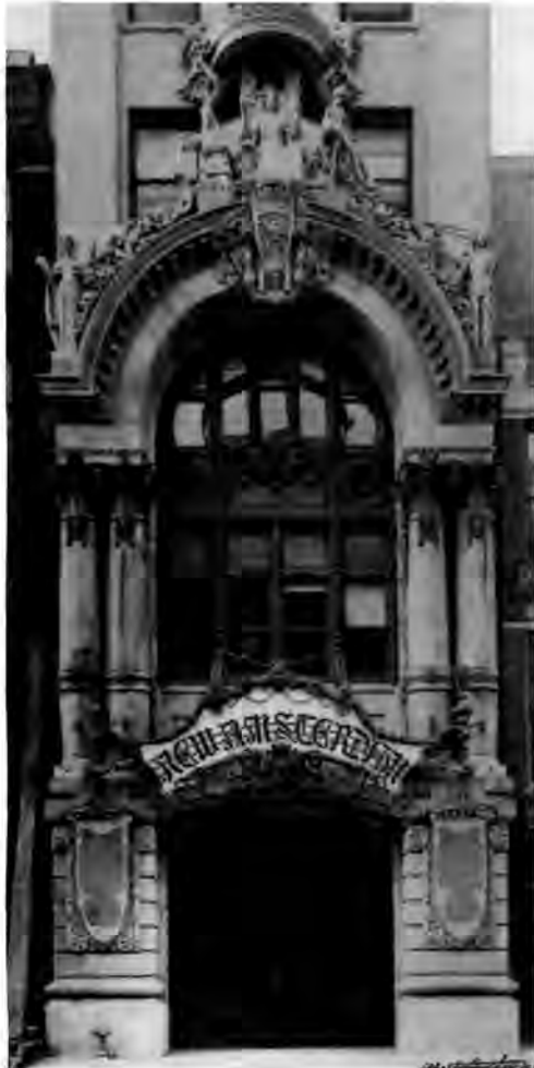
The highly decorative, Art Nouveau style New Amsterdam Theater in New York City is one of the gems of Times Square. It is being rehabilitated using the historic preservation tax incentives. Photo courtesy Museum of the City of New York.
