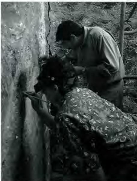
approximate ratio of 1:3.<sup>2</sup> Examination of the samples under the microscope revealed a three layer plaster system, with a thick, single coat of plaster applied directly on the masonry, and at least two campaigns of painted designs, separated by multiple layers of limewash.
