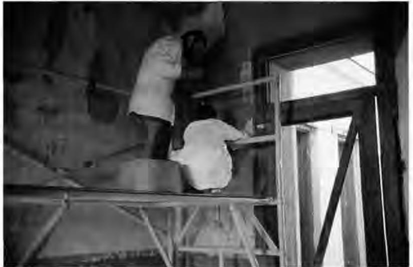
cases where removal would seriously compromise the historic plaster. It was replaced with more sympathetic material made of hydrated hydraulic lime and sand. Deep losses within the plaster body were filled with edging material and recessed approximately 1/8" below the fragment surface. Shallow fills and open cracks were filled with a mixture of one part hydrated hydraulic lime and three parts fine silica sand.
