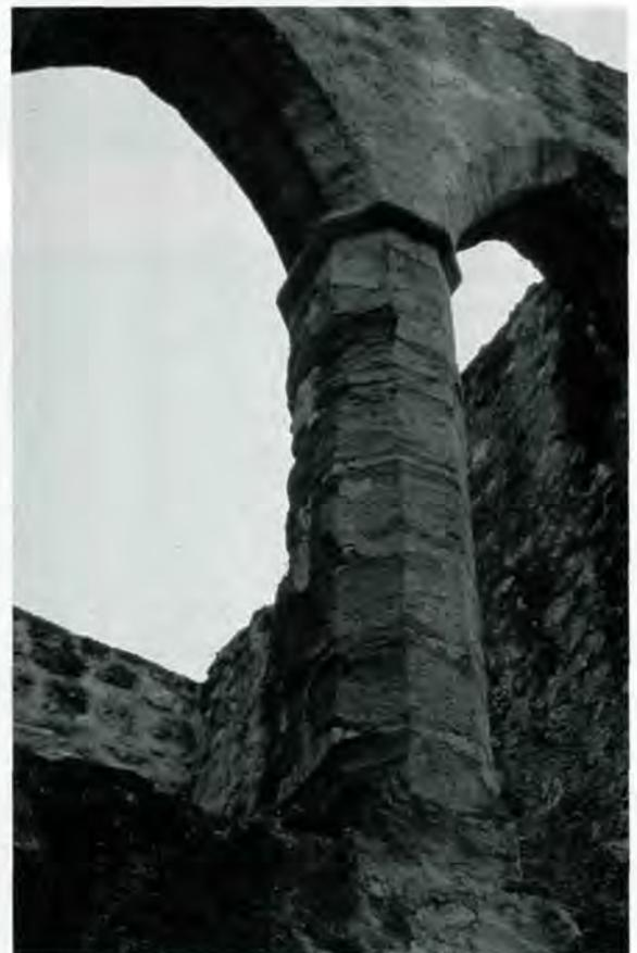
structure were retained, but the internal partition walls were demolished and replaced. All of the new masonry was laid in lime mortar, with the exception of the drums of an octagonal column, which were laid in gypsum mortar. These rebuilt elements of the convento were meant to serve as interior spaces, with the column accenting the second story of a stair hall; however, in 1868 the
