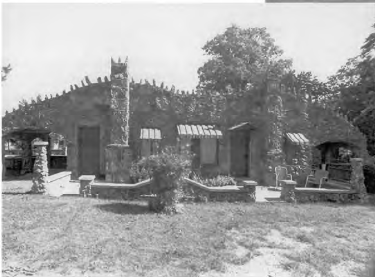
Built around the opening to the cave that shelters the largely underground Crystal River, the imaginative buildings of the 1934 Crystal River Tourist Camp, Cave City, AR, are described as mason Prince Matlock's "Mannerist" interpretation of the organic rustic style of automobile tourist camp. Photo by S. Mitchell, Arkansas Historic Preservation Program.
