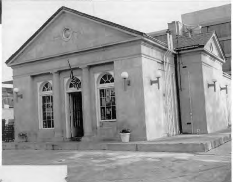
The Embassy Gulf Service Station, Washington, DC, was designed in a Neo-Classical mode as an example of "artistic" stations intended as miniature civic monuments. Because of its location, this design by architect Pierre L.R. Hogner was subjected to the design review scrutiny of the Commission of Fine Arts and the National Capital Planning Commission. Photo by Tracerics.
