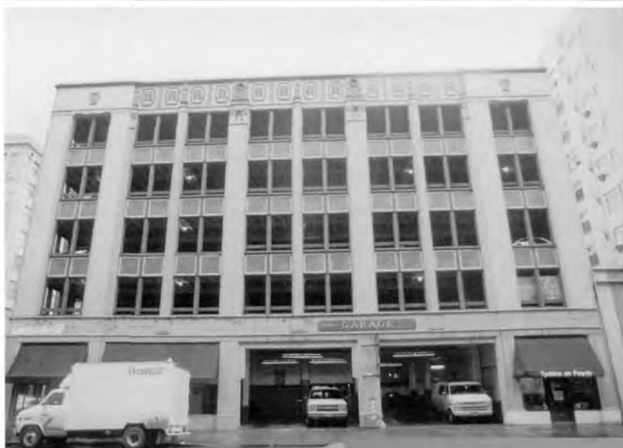
In response to the dramatically increased demand for automobile parking in the downtown central business district, the Imperial Garage, Portland, OR, was built in 1923 as the city's first multi-floor parking garage constructed specifically as an automobile parking garage. Photo by John M. Tess, Heritage Investment Corporation.
