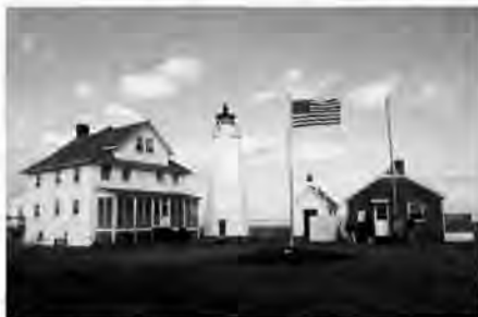
Cove Point Light Station, near Lusby, MD. Tower constructed 1828. Photo by Candace Clifford.
