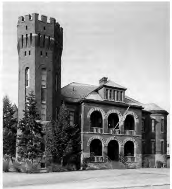
Hudson Armory (c. 1898), Hudson, NY. 1930s photo courtesy Tom Duclas, Curator, NYSDMNA.
