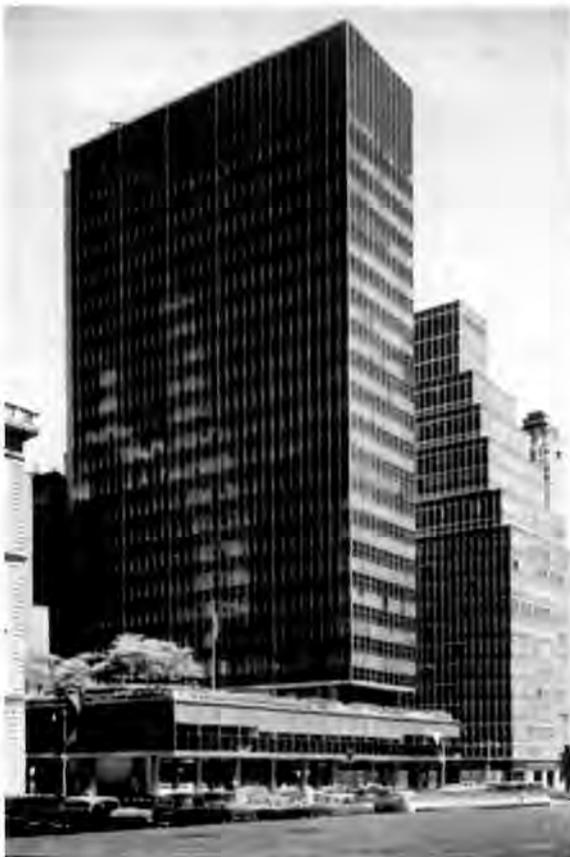
Fig. 3. An early aluminum curtain wall used in conjunction with the then more traditional limestone curtain wall. The fluted aluminum spandrel plates and center pivot windows have contributed to water leakage over the years.
