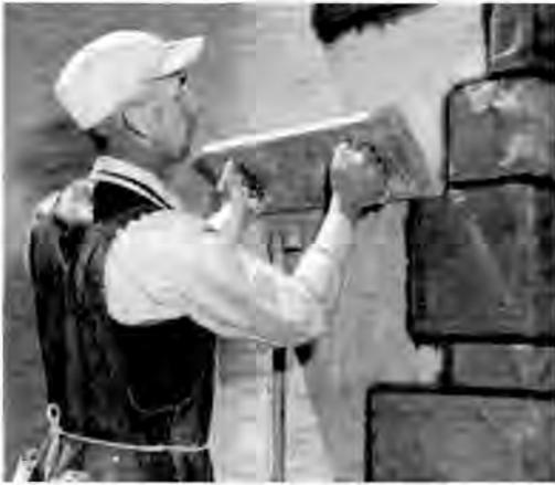
was "moulded in dies cast from selected quarry stone." As with other products, pigments were used to match the desired stone color.
