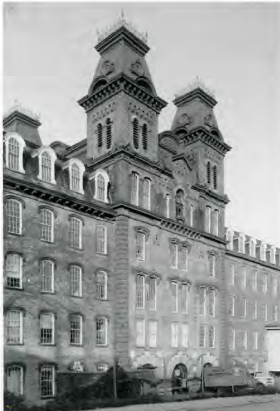
Harmony Manufacturing Co. Mill No. 3, central block, west face; quoins are cast iron. Photo by Jack E. Boucher.
