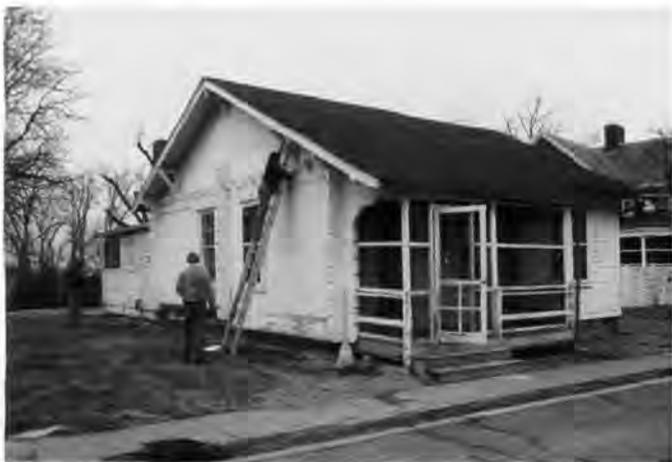
A risk assessment of the property is recommended when lead-based paint is present. The paint's location and condition should be recorded and a list of priority risk areas should be identified. Deteriorated paint and friction surfaces on windows and doors should be treated first.
