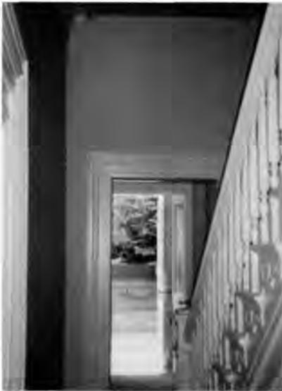
Some residential properties scheduled for full hazard abatement may require a greater level of paint removal or encapsulation than non-residential properties. In this instance, loose deteriorated paint was wet sanded and then the trimwork was painted with several thin layers of a special encapsulant paint coating.
