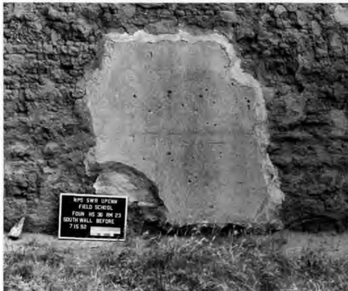
Fig. 7. Mechanics Corral (HS 36), Room 23, Fort Union. Plaster fragment before recent conservation. Note unsightly and failed previous edging.
