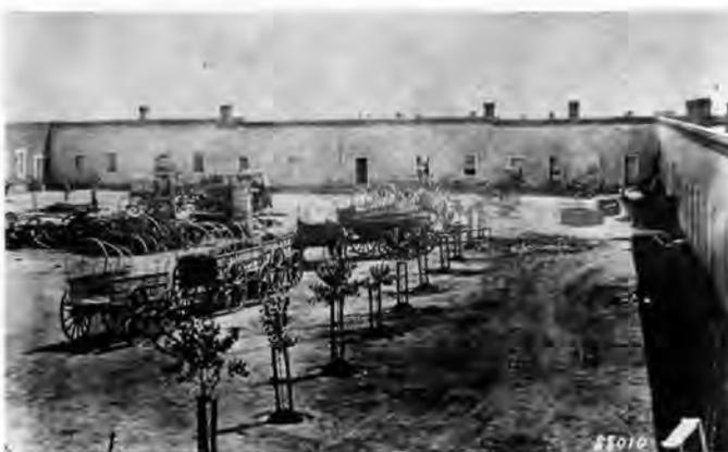
Fig.5. Mechanics' Corral, interior, 1866. Note fresh exterior plaster up to the brick cornice.
