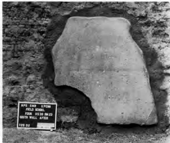
Fig. 8. Mechanics Corral (HS 36), Room 23, Fort Union. Plaster fragment after recent conservation. Note new edging flashed into adobe wall.
