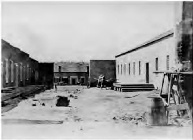
Fig.4. Quartermaster Storehouse loading yard, c. 1866. Note plastering in progress on the right wall.
