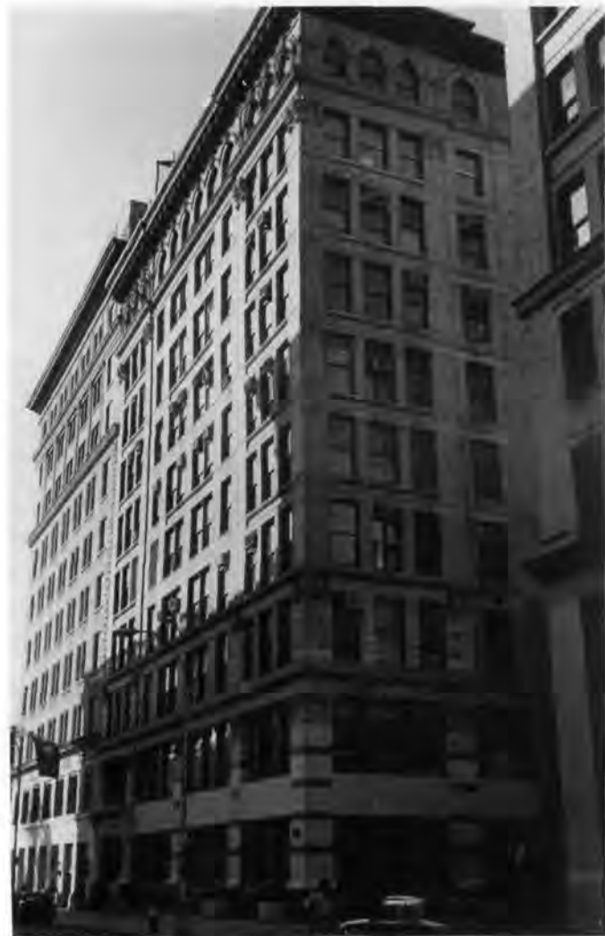
Triangle Shirtwaist Factory Building (Brown Building), 23-29 Washington Place, New York, NY. Photo by Andrew S. Dolkart, 1989.
