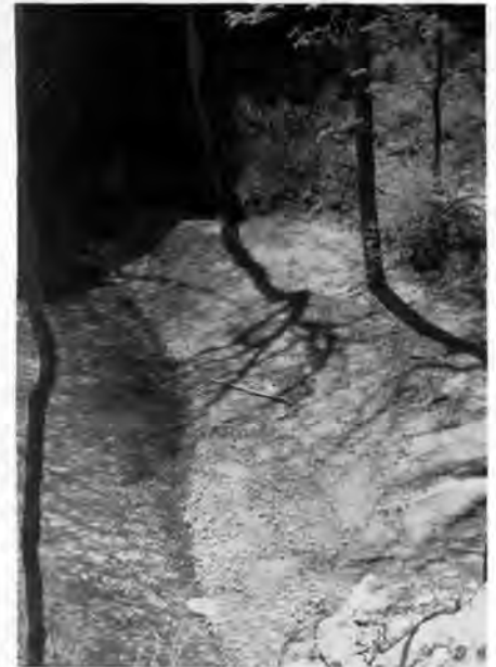
Fig. 4. View of completed bulwark. Compare with Fig. 1. Notice reconfiguration of the stream and position of the two large trees. Cave entrance is in the upper left-hand corner of the photo.
