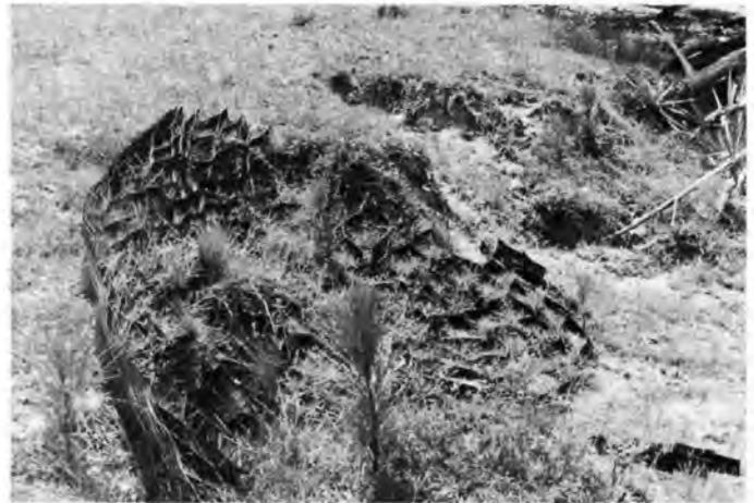
Fig. 7. GEOWEB place in animal trail along cutbank. Note pine seedlings.
