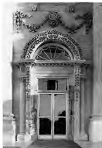
Photograph of the north entry door, stripped of the 32 coats of paint that had occluded the stone carving. Photo by Jack E. Boucher, 1989, HABS.
