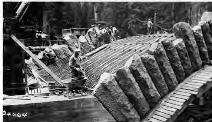
Original Bureau of Public Roads construction reports provide HAER researchers with details of the building process from excavation to completion and offer pictorial evidence of construction technologies and labor practices. Construction of Deer Creek Bridge in Mount Rainier National Park, 1939.
