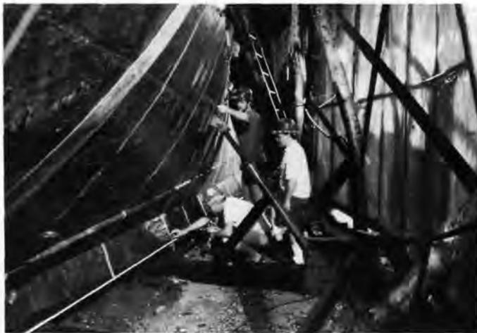
*Snow Squall* project director David Switzer, maritime intern Karl Bodensiek, and HAER Architect Dale Waldron (from left) attach station lines to the bow section of the clipper ship in preparation for measurement of the hull's starboard side curvature. Photo by Molly Horvath, 1992.
