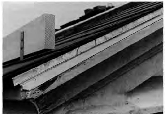
6. Cypress, a durable wood, was selected for the snow boards and stainless steel was selected for the support brackets because it will not corrode. Note the lead coated copper drip edge under the slate and the slight kick-up at the eave created by a cypress wood spacer. The deteriorated portion of the cornice was in the process of being repaired.
