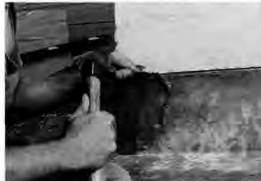
3. Traditional methods were used to pack lead wool into flashing reglet (narrow slit) joints to hold the cap flashing tight with the stuccoed chimney.
