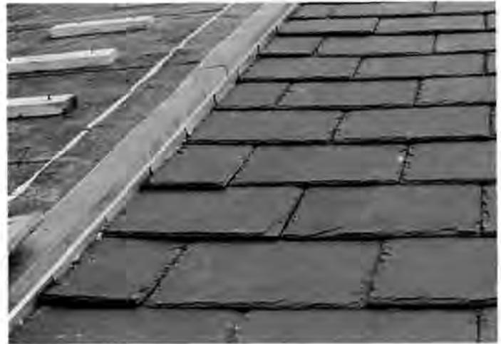
2. Modern methods of detailing joints were used where moisture could penetrate to the roof deck. At this offset between the lower portico roof and the main block, a hidden rubberized membrane was selectively used in connection with traditional lead-coated copper flashing.
