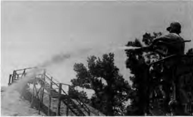
Photograph showing hydroseeding of Santee Indian Mound in progress. The sprayer mounted on the truck was used on the front side of the mound and a hose was used to reach the top, sides and back.
