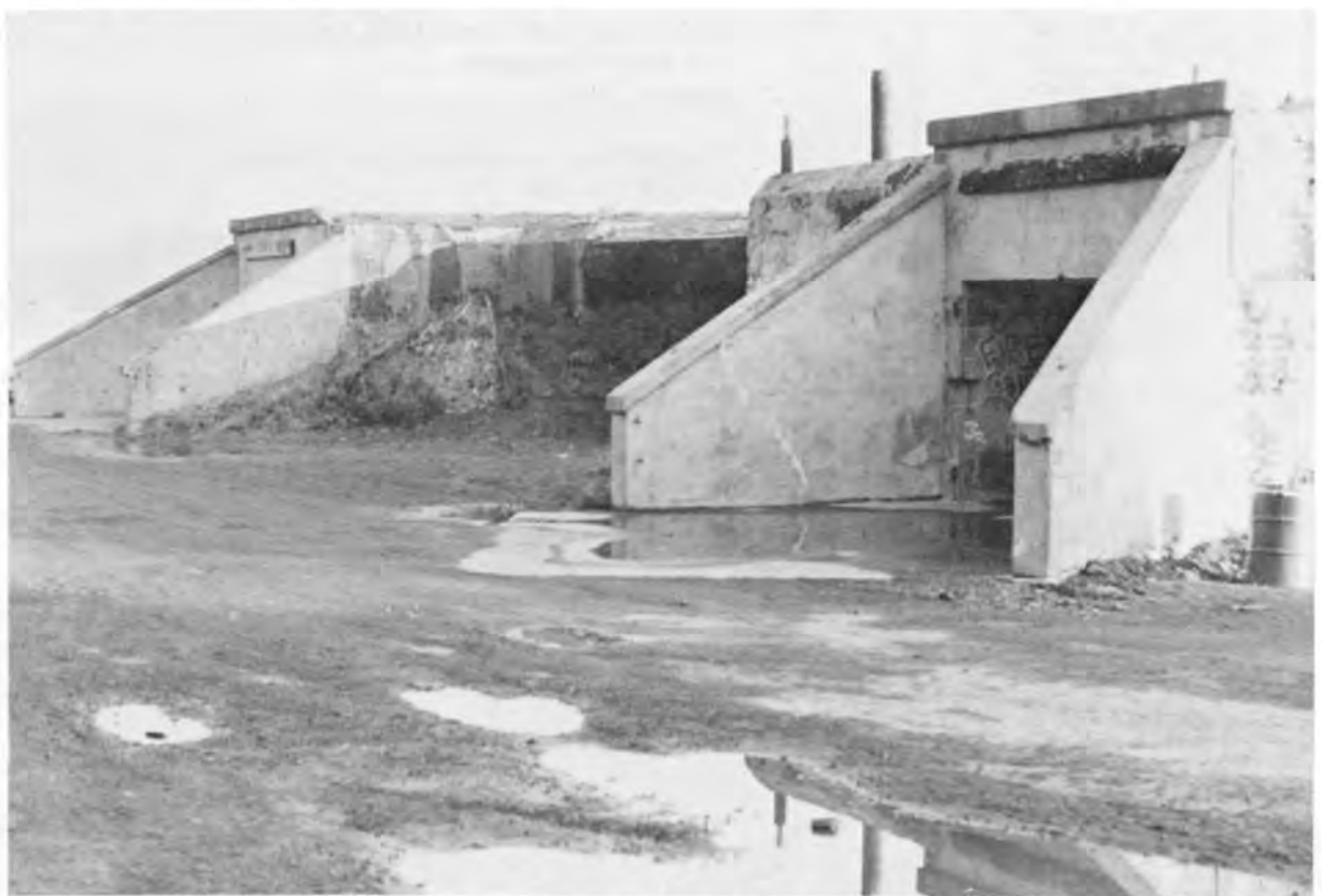
Casemated magazine at 8-inch gun battery of Fort Abercrombie, a subpost of Fort Greely, Alaska. This rear view shows the two entrances to a U-shaped passage. NPS photo by Erwin Thompson, 1983.
