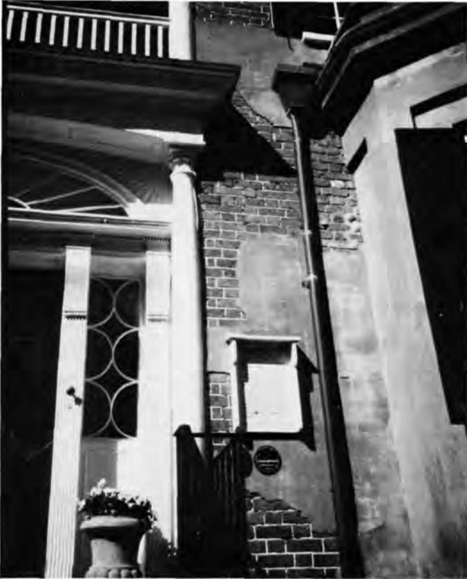
9. The existence of such fine quality mortar joints is evidence that this brick house in Charleston was not stuccoed originally.
