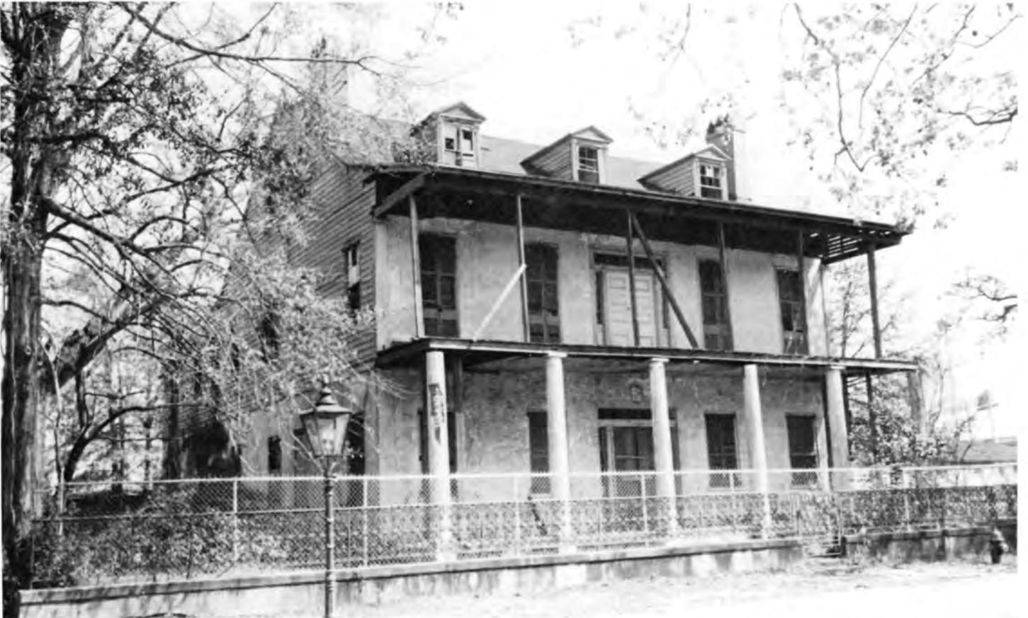
20. The primary facade, and first story of the side elevation of this early 19th century house in Mobile have been stuccoed and scored, but the second story of the side elevation is clapboarded.
