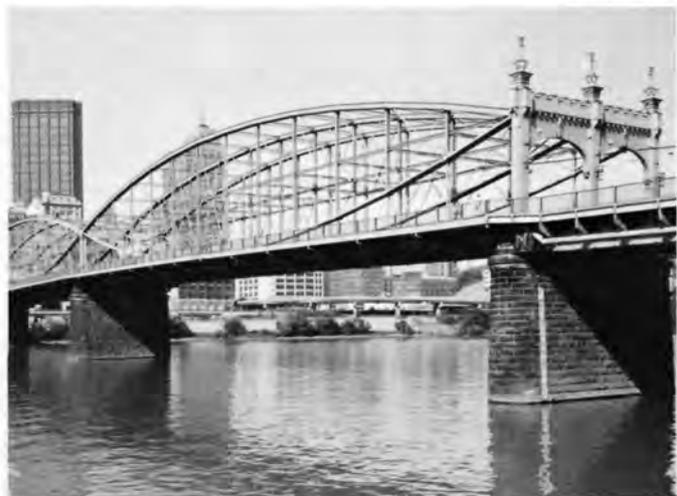
Smithfield Street Bridge (1883, 1891). Designed to span the Monongahela River in Pittsburgh by Gustav Lindenthal, one of America's most prominent bridge engineers, this is the oldest steel-truss bridge in the country. It is scheduled to be rehabilitated for continued vehicular use. Photo by Jack E. Boucher for HAER, NPS.
