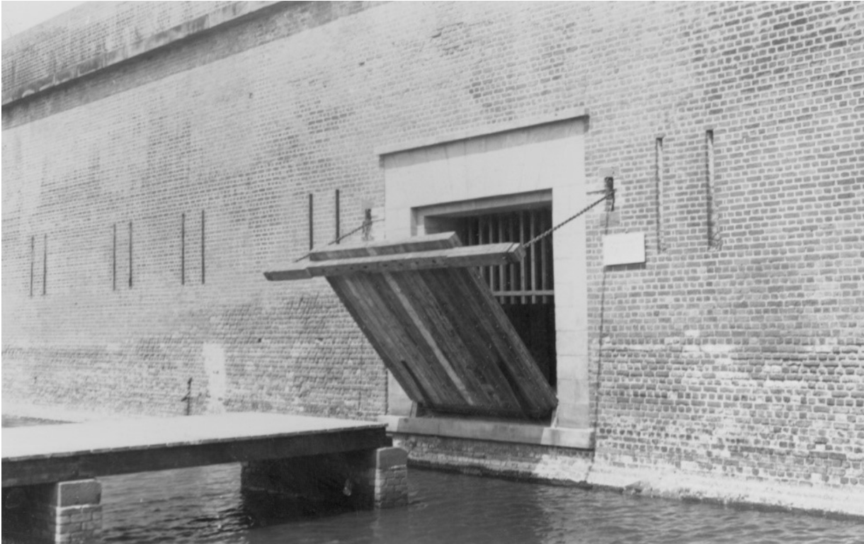
The drawbridge being raised in the 1960s.
