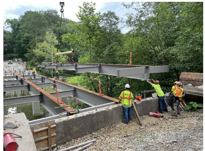
Crews installing steel girders for the Yorktown Creek bridge.
