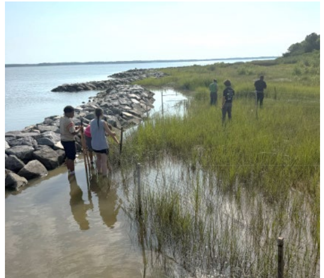
Park staff repairing fencing around cordgrass plantings.
